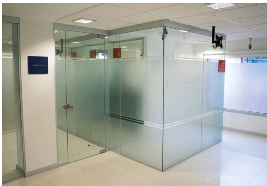
Safety protective partitions in Banco Galicia, Branch No. 391 - Cañuelas
